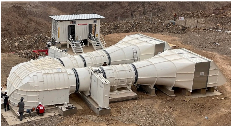
Project in north Africa with a plenum, dampers, single stage fans, baffles & electrical container
